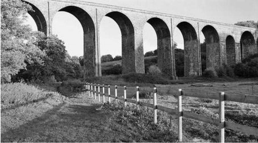
The Pensford Viaduct
